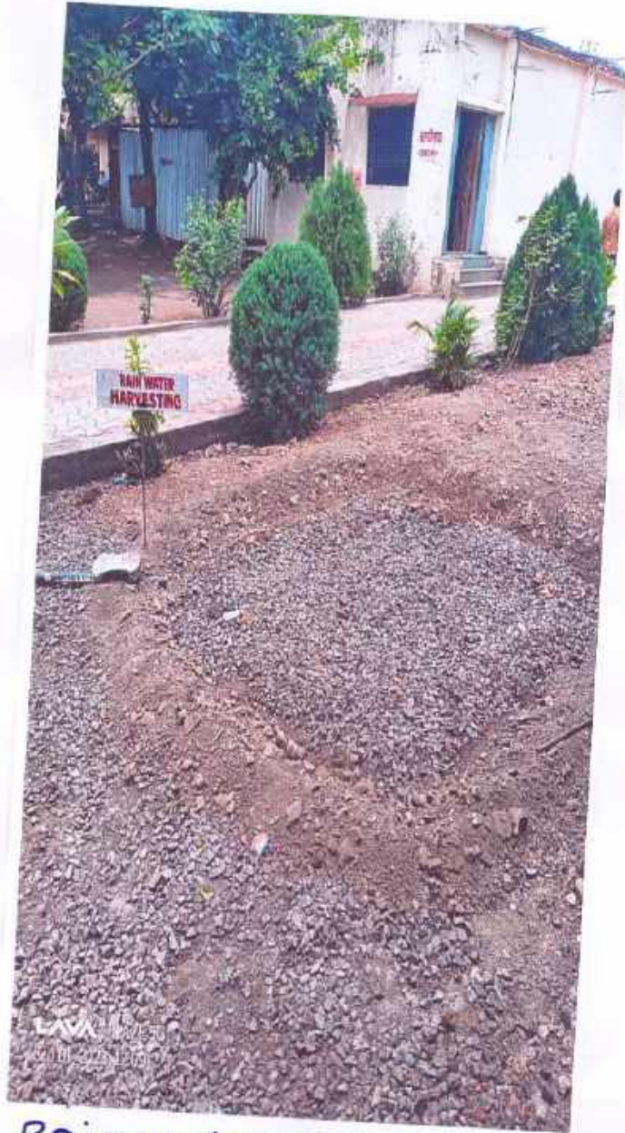
Rain Water Harvesting
